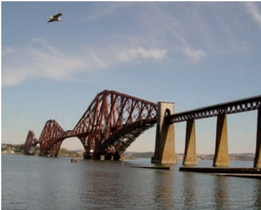
Vista general del puente del Firth of Forth.
